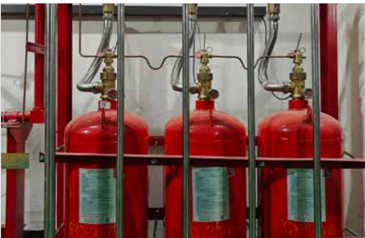
HFC-227ea (or FM200) Automatic Fire Extinguishing System at Jinmao Plant 1 of Elite Electronic Material (Kunshan)
