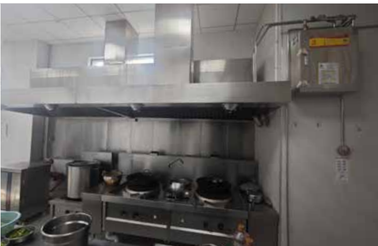
Automatic kitchen fire suppression system at Elite Electronic Material (Huangshi)
