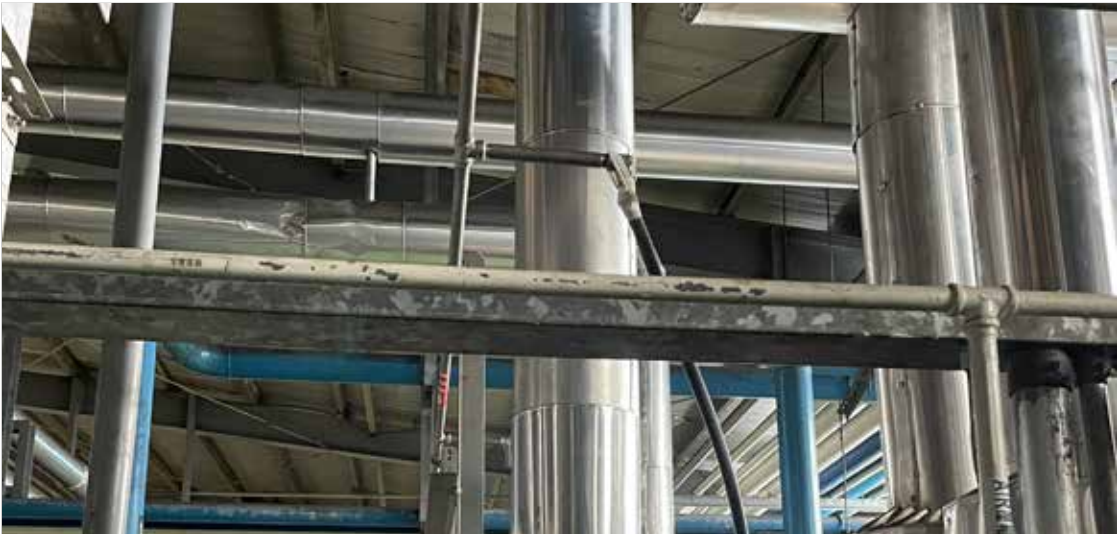
A water mist fire suppression system was installed in the heat transfer oil pump area
